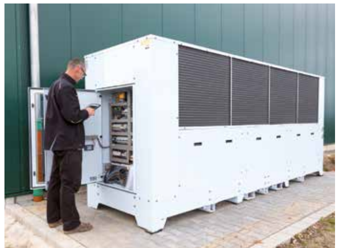
On site commissioning
